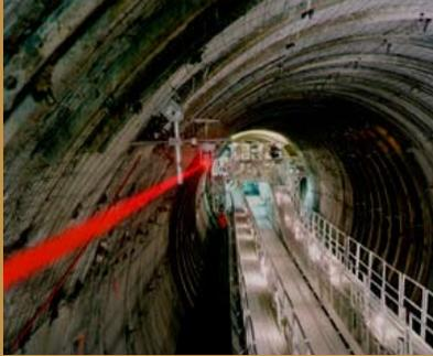
View of the rear of the tunnel boring machine showing the laser guidance system in operation.
