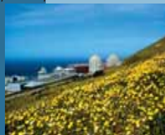
The Diablo Canyon nuclear power plant in California
